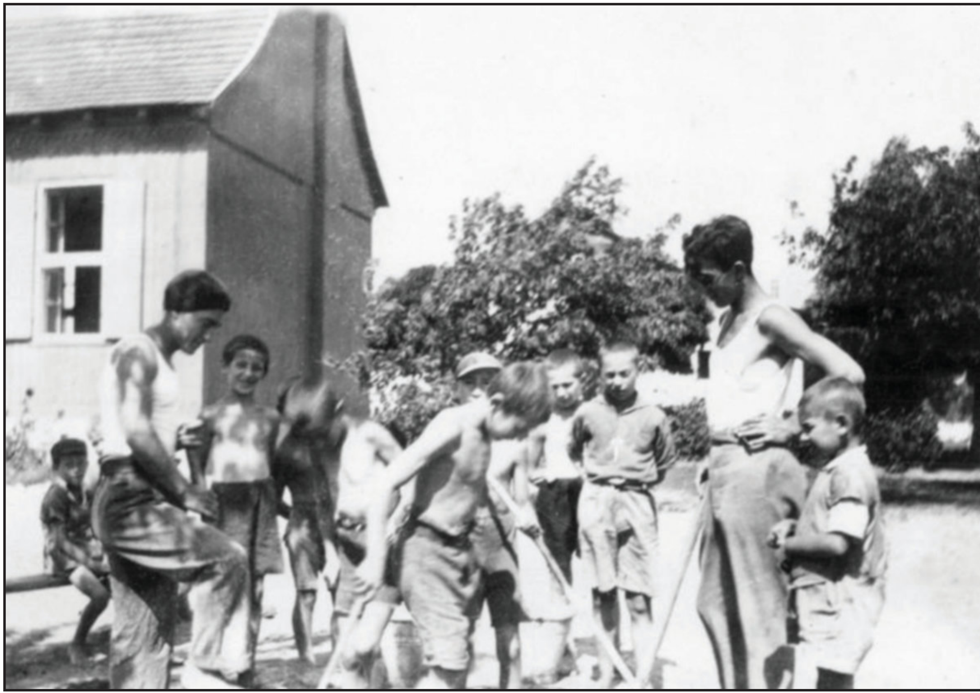
Paving the paths between the bungalows at the summer camp. Photographed by Shlomo in 1934.
