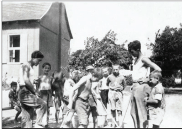
Paving the paths between the bungalows at the summer camp. Photographed by Shlomo in 1934.
